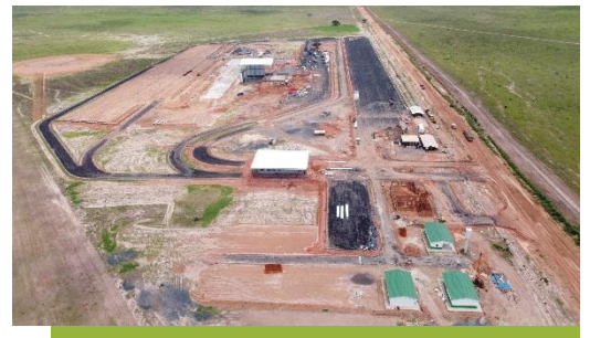
Constructions in Progress
