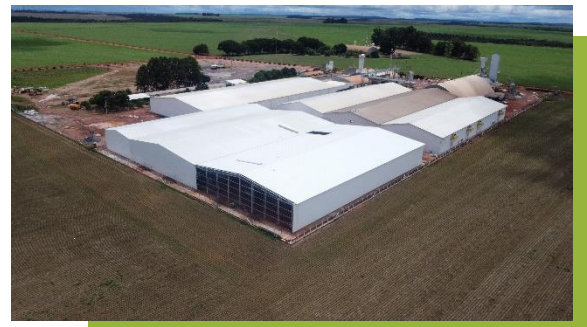
Construction in Progress / In Conclusion
