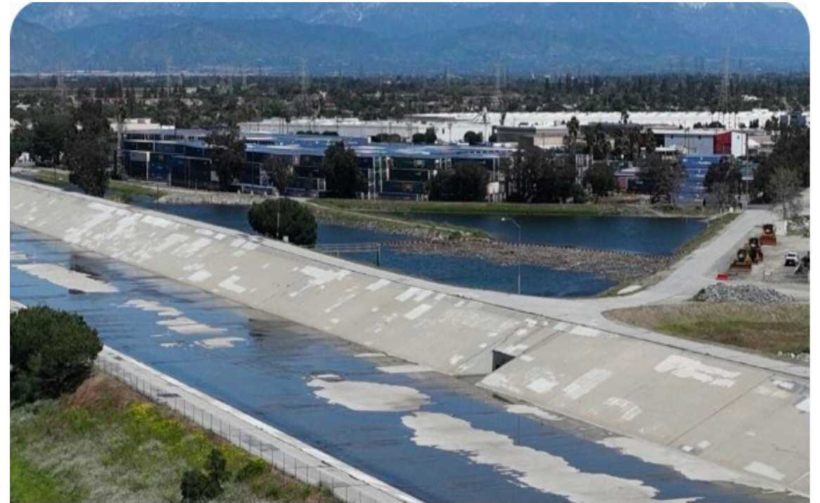
Despite historic rains in 2023, aquifers deep beneath L.A. area remain depleted
