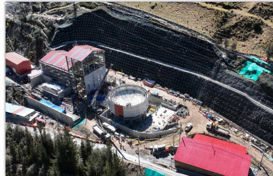
Cerro Pasco Integration Project: view of the Tailings Pumping System construction site, including the Tailings Thickener and Pump Station.
