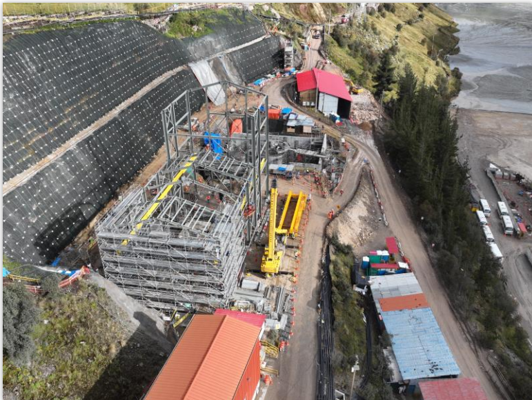
Cerro Pasco Integration Project: Aerial view of the Tailings Pumping System construction site, including the Tailings Thickener and Pump Station.
