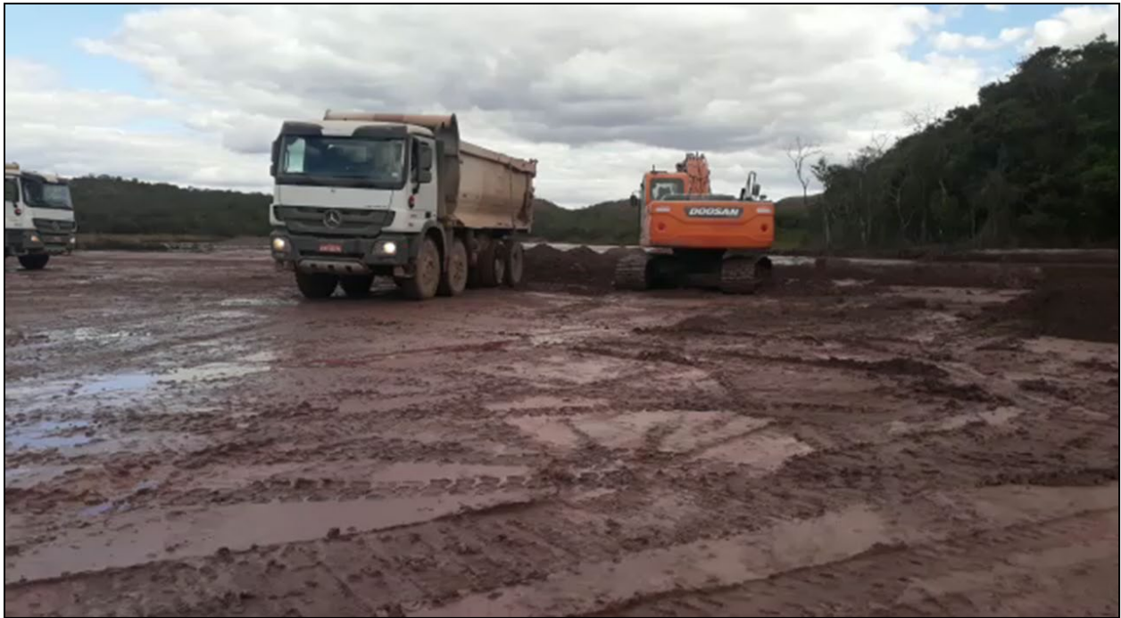
Figure 11-66: Excavation of the Aroeira Tailings
