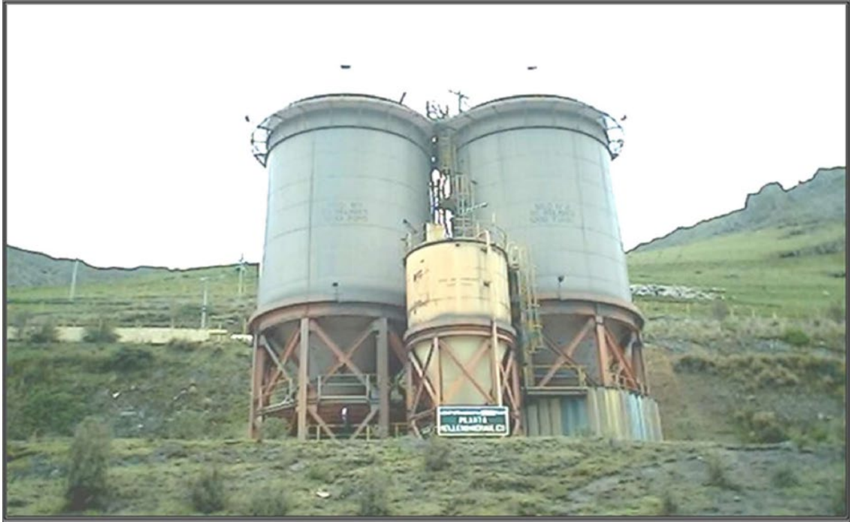
Figure 13-17: Hydraulic Backfill Plant
