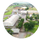
PLANT I CORN PROCESSING: 24,000 t/month
