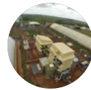
SOYBEAN PROCESSING PLANT: 1,500 t/day
