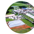
PLANT I SOYBEAN PROCESSING: 1,700 t/day
